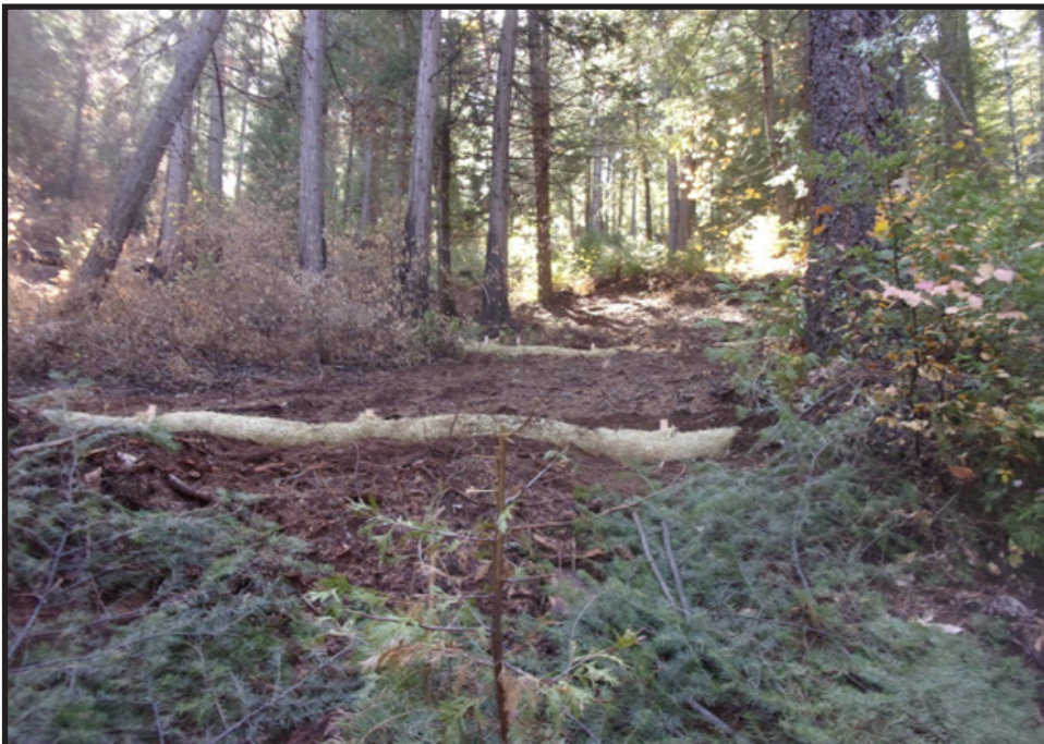
Two lines of wattles installed on fire dozer line November 2021
